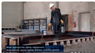
Application of concrete release agents
